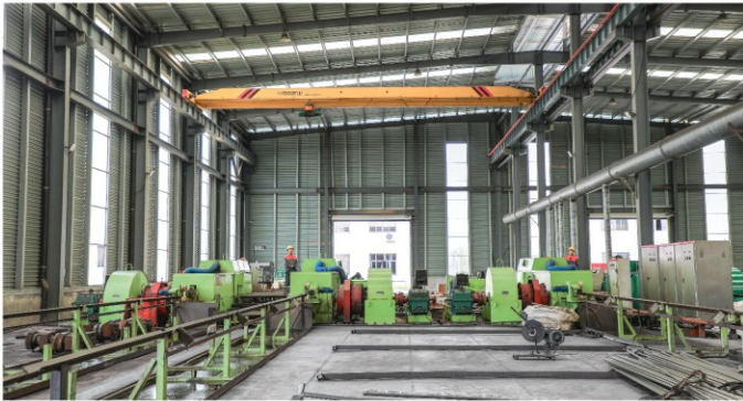
冷轧车间 Cold-rolling Workshop
